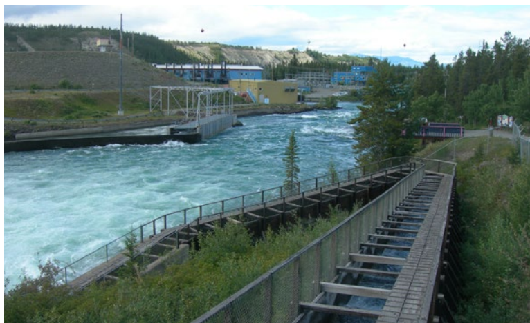
A wooden fish ladder allows salmon to make their way upriver around the Whitehorse dam and hydroelectric plant in The Yukon, Canada. Photo by Jimmy Emerson, DVM via Flickr. License
