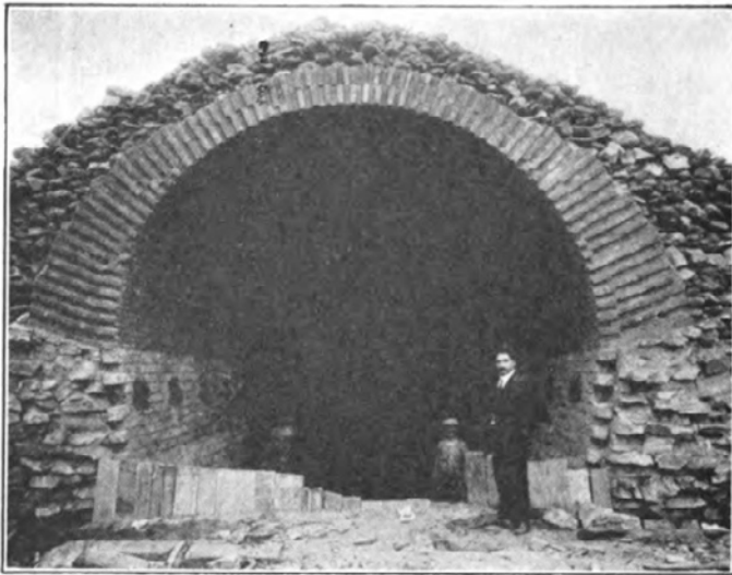
Above: A section of the Wingohocking Creek sewer 17 feet in diameter. Photo taken in 1913. From Michael McShea, phillyandstuff.blogspot.com
