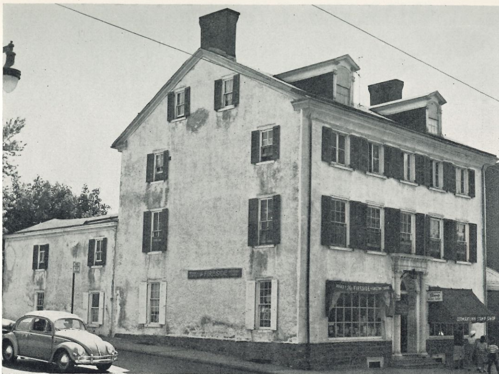
The Shippen-Blair House before renovation. Photograph courtesy of the Philadelphia Historical Commission.
