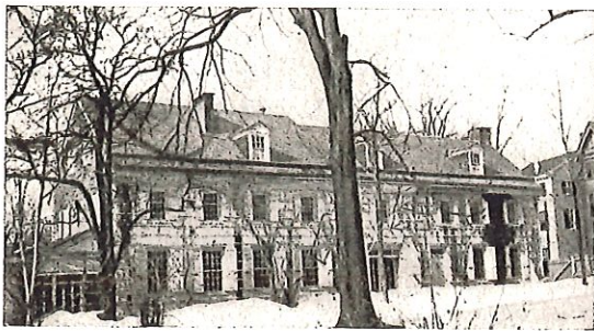
Wyck—oldest house in Germantown
